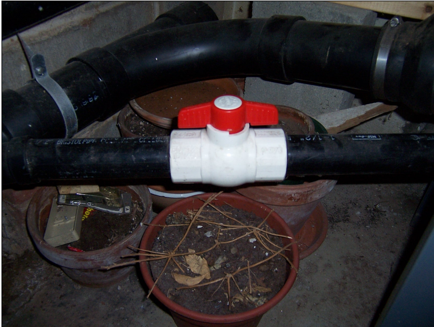
Figure 2: ABS drain valve to be removed and replaced with PVC valve
