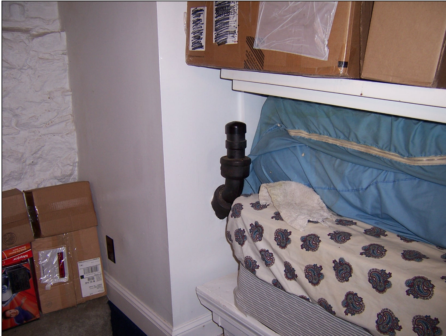
Figure 10: Original drain location cut and capped
