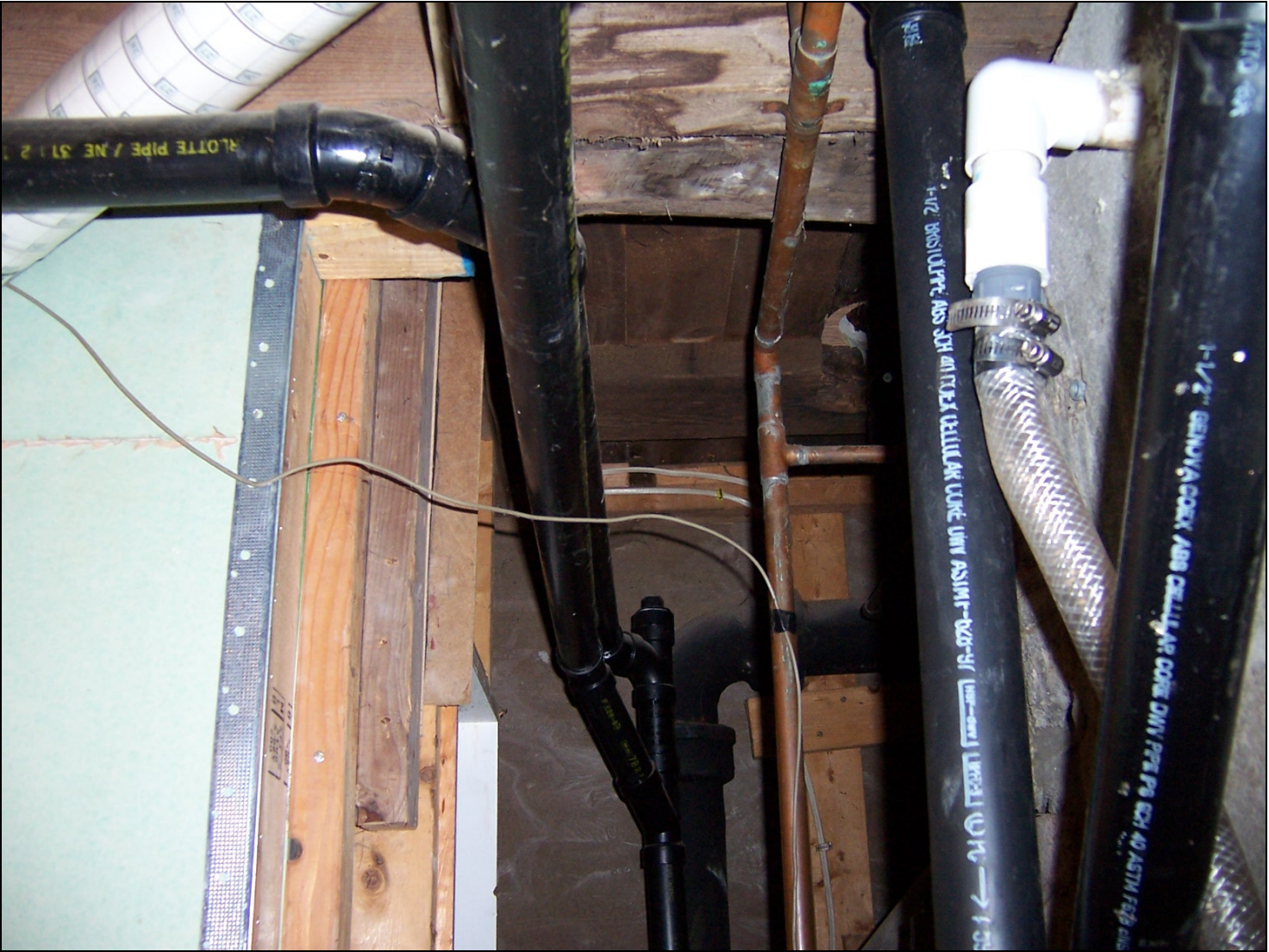
Figure 7: Drains stacked above each other
